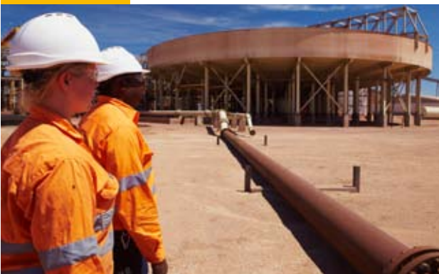
The Prominent Hill processing plant
