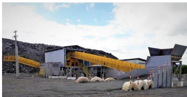
Figure 11: Antas ore sorter installed
